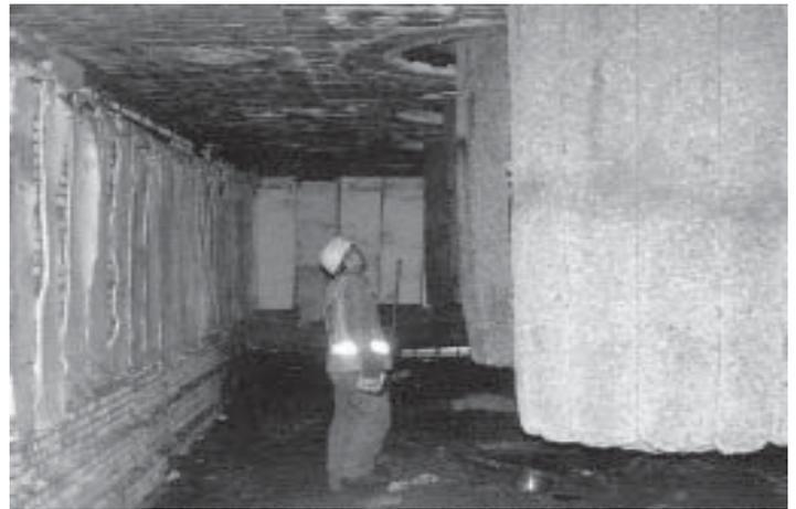
*A final check of Melter 1 before recommissioning.* improved taphole cooler blocks, thicker wall refractory with tongue and groove construction, thicker roof refractory, improved refractory materials, much larger springs and tie-rods, considerably stronger end-wall structural beams, and much stronger water cooled roof beams.
