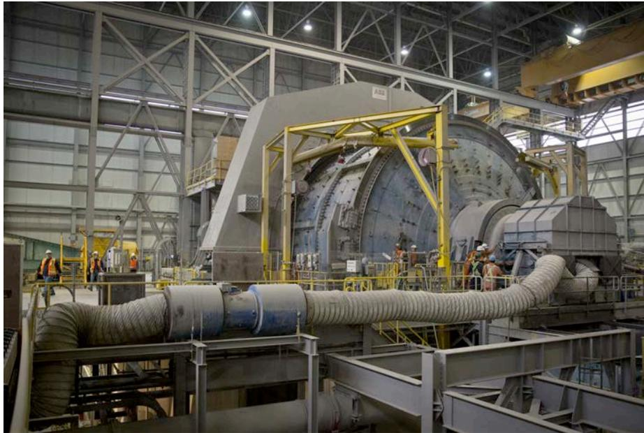
Figure 6 – Exhaust fan connected to the discharge trommel
